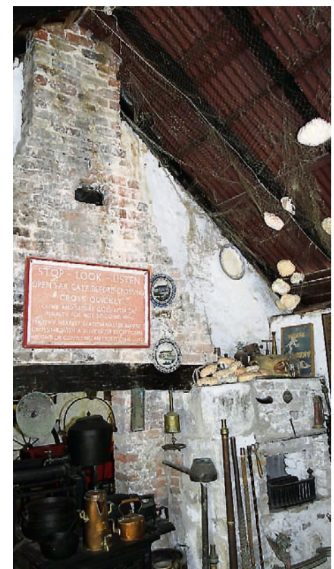
The oven and chimney inside the original kitchen at Greenwood Great House.
