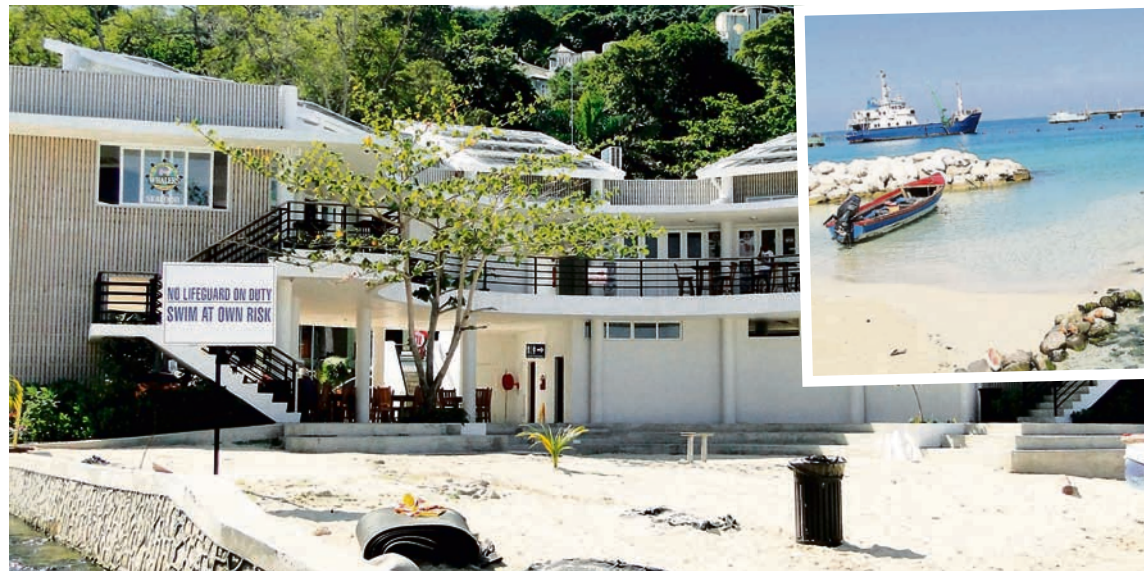
Another section of the new concrete structures in the Ocho Rios Fishing Village.
