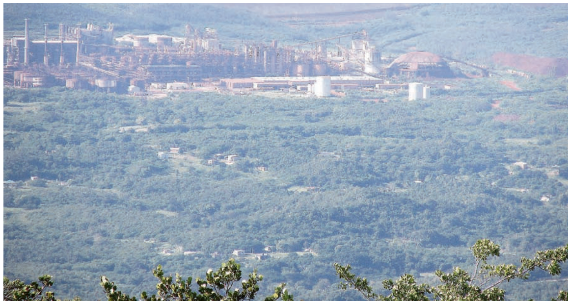
A bauxite plant in south St Elizabeth from Lincoln in Manchester.
